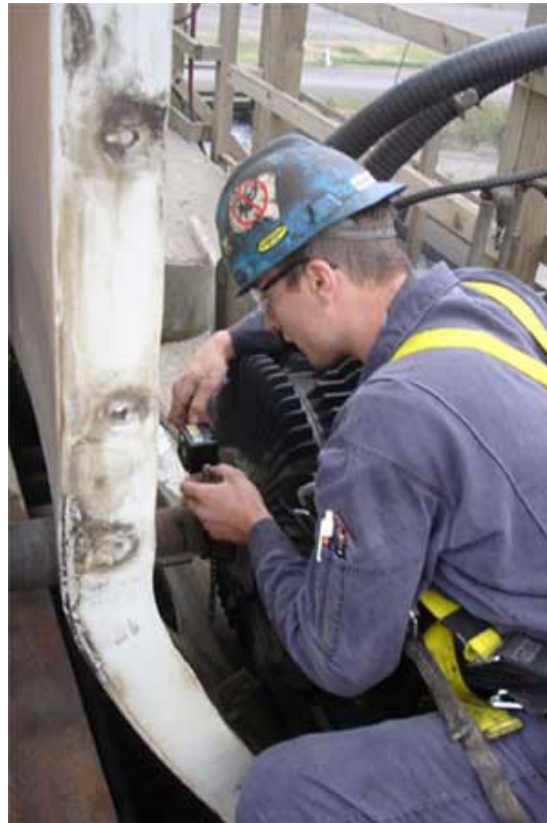
One Laser/Detector is mounted on the motor shaft which is outside the cooling tower wall.
